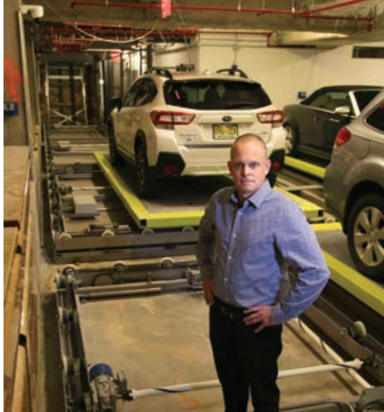
TIGHT FIT: Nash of Gotham Parking Systems brought this 5BY2 Puzzle Parking System to 152 Elizabeth St.
