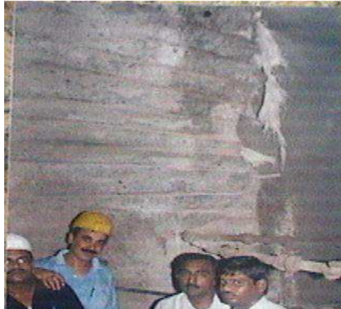
Fig. 5(b). Pier nose wall after pre-split blasting
