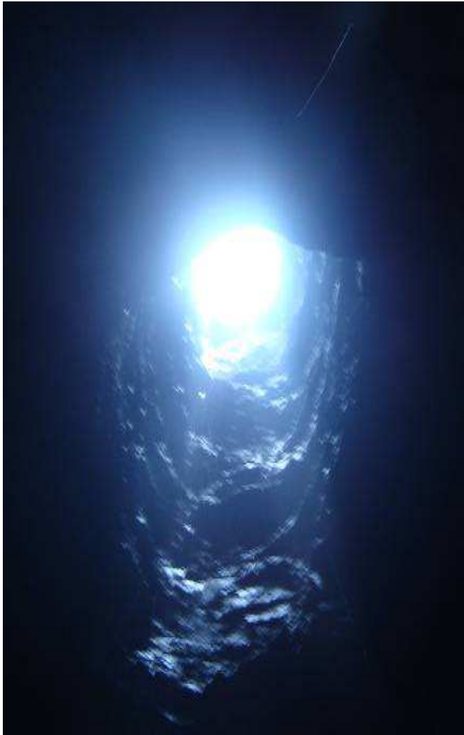
Fig. 4. Profile of pilot surge shaft excavated by long hole raise driving at Koilsagar
