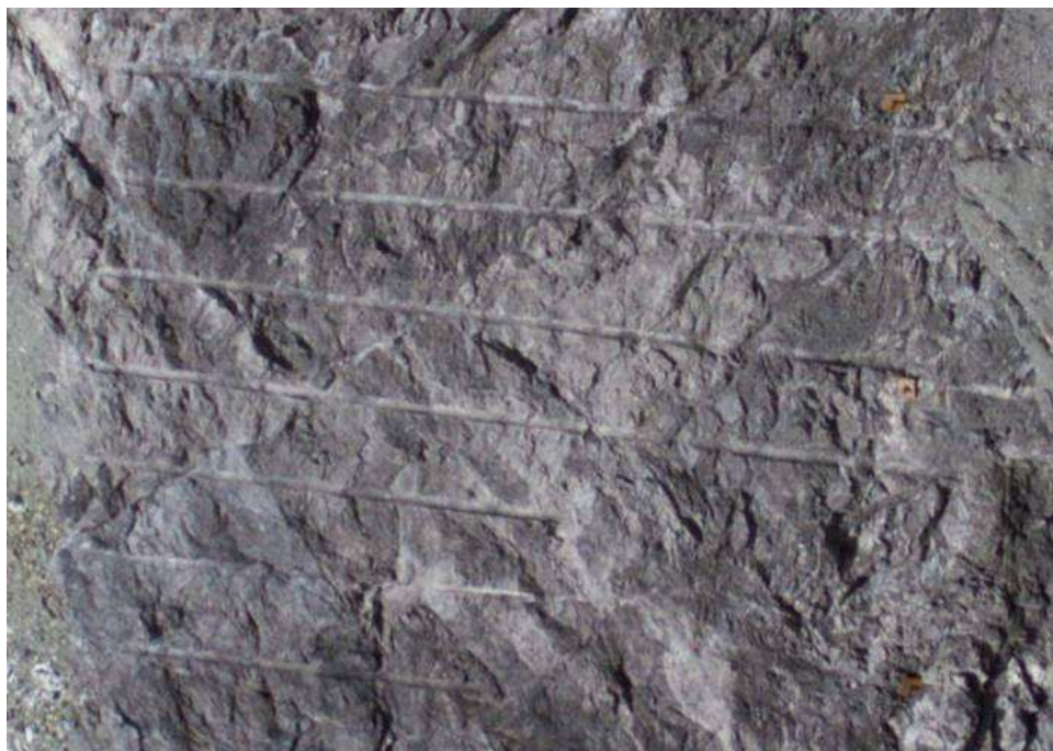
Fig. 7. Improved blast performance of smooth blasting in the form of smooth profile at KHEPP
