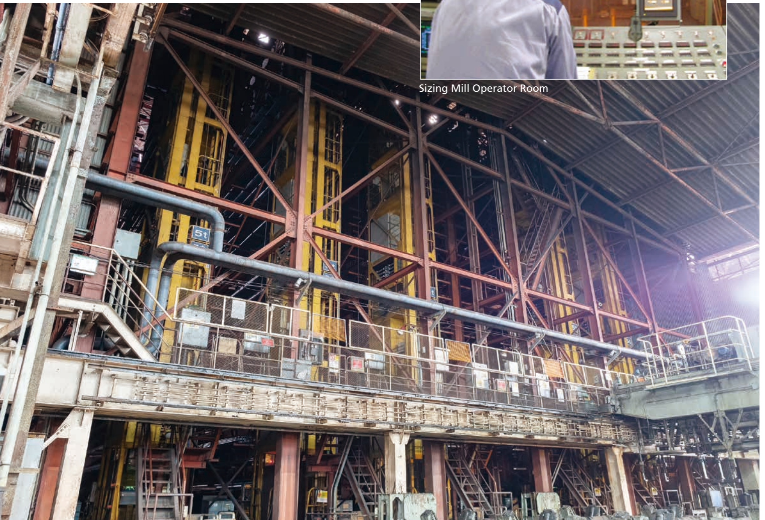
Automatic Rack System
