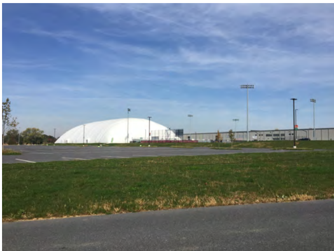
The dome at the Nook is used primarily by the USA Women's Field Hockey team and features an irrigation system to keep the surface of the playing fields uniformly wet.
