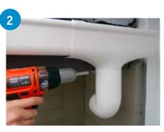
Connect downpipe bend to expansion outlet using a screw to hold bend in place. To allow easy removal for cleaning debris do not solvent cement bend to outlet.
