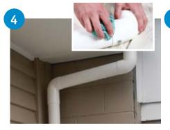
Solvent cement all remaining elbows to downpipe on ground, before completing offset installation.
