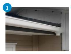
Install expansion outlet as per spouting installation instructions.
