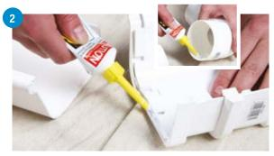
Marley solvent cement (MCS°) should be applied evenly **to both surfaces** being joined. Then press both surfaces together and hold for 20–30 seconds
