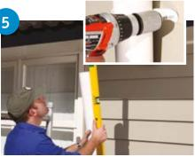
Use a level of plumb line to mark where the downpipe will sit against the wall. Ensure downpipe clips are spaced no more than 1.2 metres apart and the first clip is a maximum of 200mm below the downpipe bend. Downpipe clips to be secured with two stainless steel screws.
