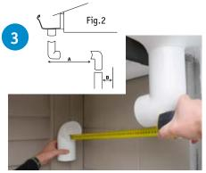
Determine the offset length (A) using Fig 2 allowing for depth of socket and taking into consideration the downpipe bracket distance from the wall (B). Cut downpipe as per measurements.
