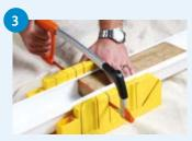
Cut replacement section on ground and solvent cement a joiner and expansion joiner to each end.
