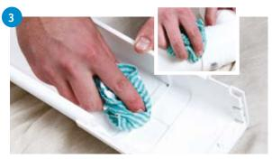
Any surplus solvent cement should be removed immediately with a damp, clean, lint free cloth. Leave sitting for 10 minutes.
