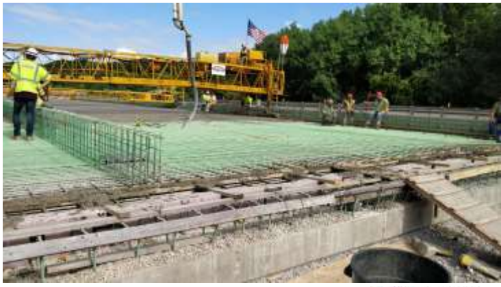
Construction of the bridge deck
