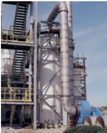
A packed bed condenser recoups energy by cooling and condensing water evaporated in the spray dryer to heat process water needed in the facility.
