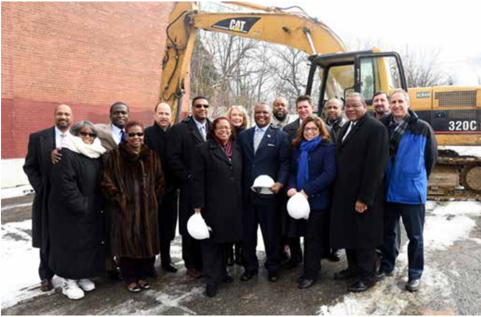
County Executive Rushern Baker, III joined community leaders and the Landex Companies for a demolition party at the site of the Northeastern Supply building. Landex was chosen to develop the $36 million mixed-use facility that will include apartments, artist studios, and retail space.
