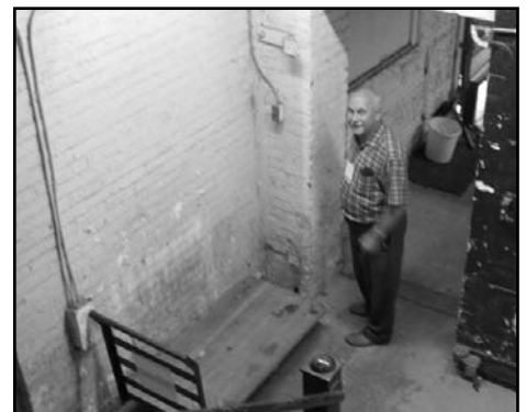
Stan Beilski inspecting the interior of the Wurlitzer factory building.
