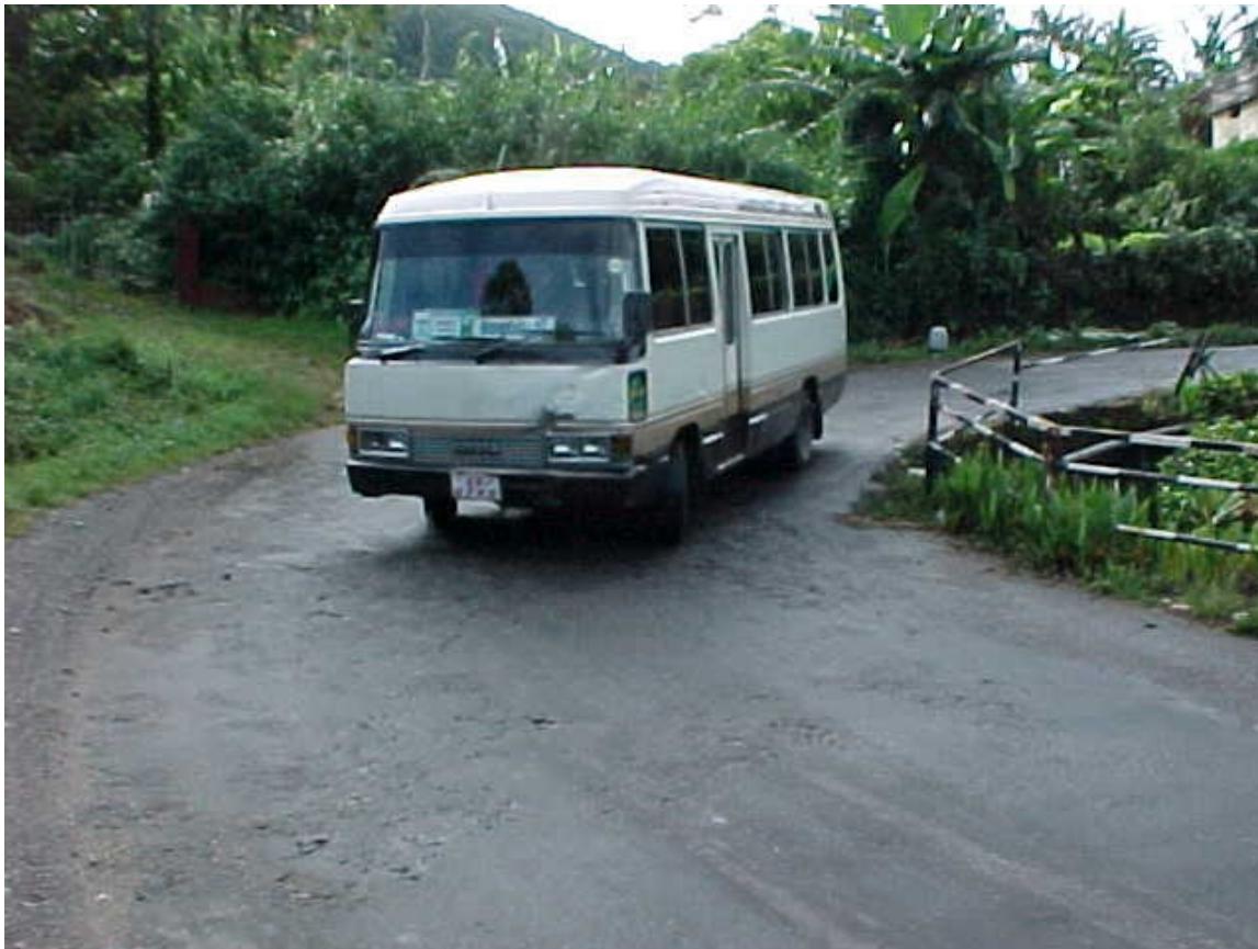
Figure 5-6. Typical Turn and Culvert on Highway 7
