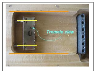
Figure 2.6 Tremolo claw Alignment
