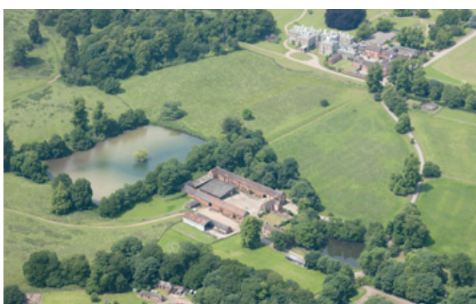
This regular courtyard farmstead was created as a model farm within Enville Hall landscape park circa 1747-8 and is attributed to the architect William Baker. It is typical of those architect-designed farmsteads associated with landed estates which are particularly to be found within south western Staffordshire. Photo © English Heritage NMR 27767/025
