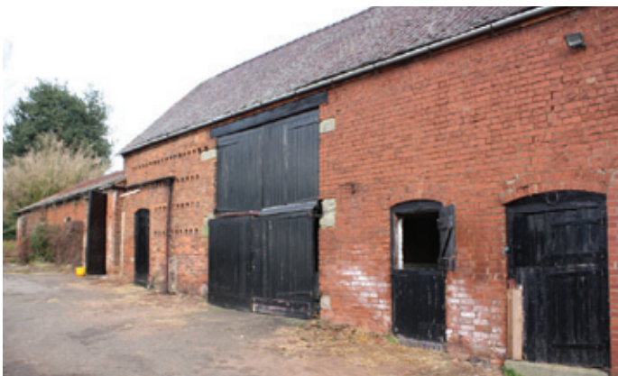
Large red brick barns are common across the lowland areas. Note the wide cow house doors to the right of the double threshing floor doors in this example of a combination barn. Photo © Bob Edwards
