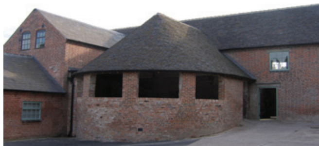
A rare example of mechanisation. This is wheelhouse which contained horse-powered machinery for threshing grain and processing fodder.
