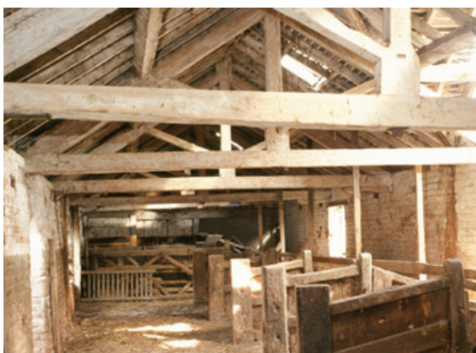
Interior of a cow house showing wooden stalls and king post roof. King post roofs made from imported softwood with iron stays and bolts comprise a standard form of roof truss used in the 19th century, most commonly from the 1840s. Photo © Mike Williams/ English Heritage
