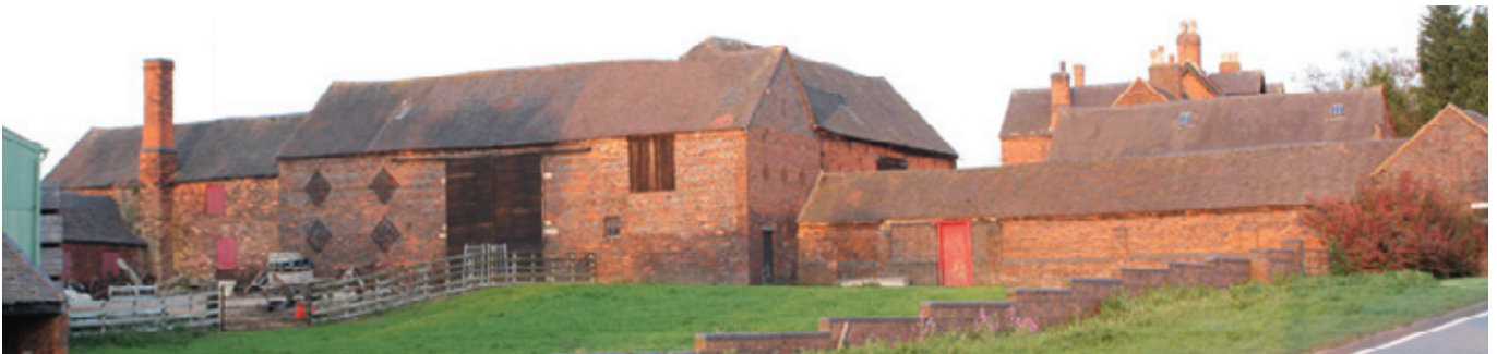
A group of traditional buildings built of brick with plain tile roofs, in the Cannock area. Note the large double doors and ventilation holes to the barn, and the chimneystack which served an engine house to the left. Photo © Bob Edwards
