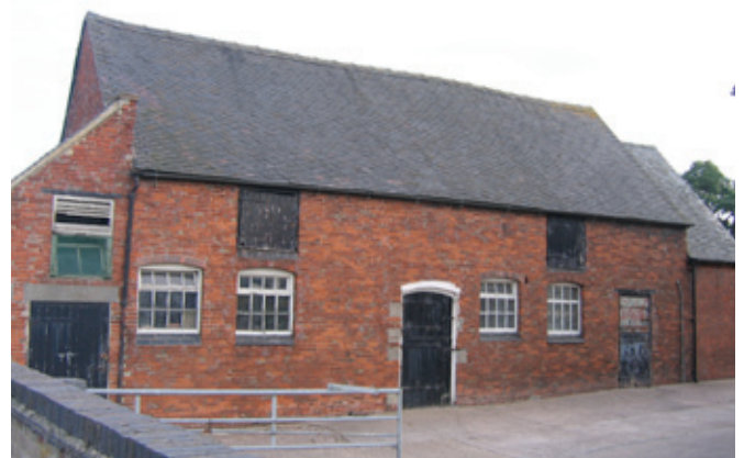
Many cow houses were converted from earlier barns and other buildings in the late 19th and early 20th centuries. The windows to this range have been inserted, and the metal frames conform to 1930s hygiene regulations for milk production. Photo © Jeremy Lake
