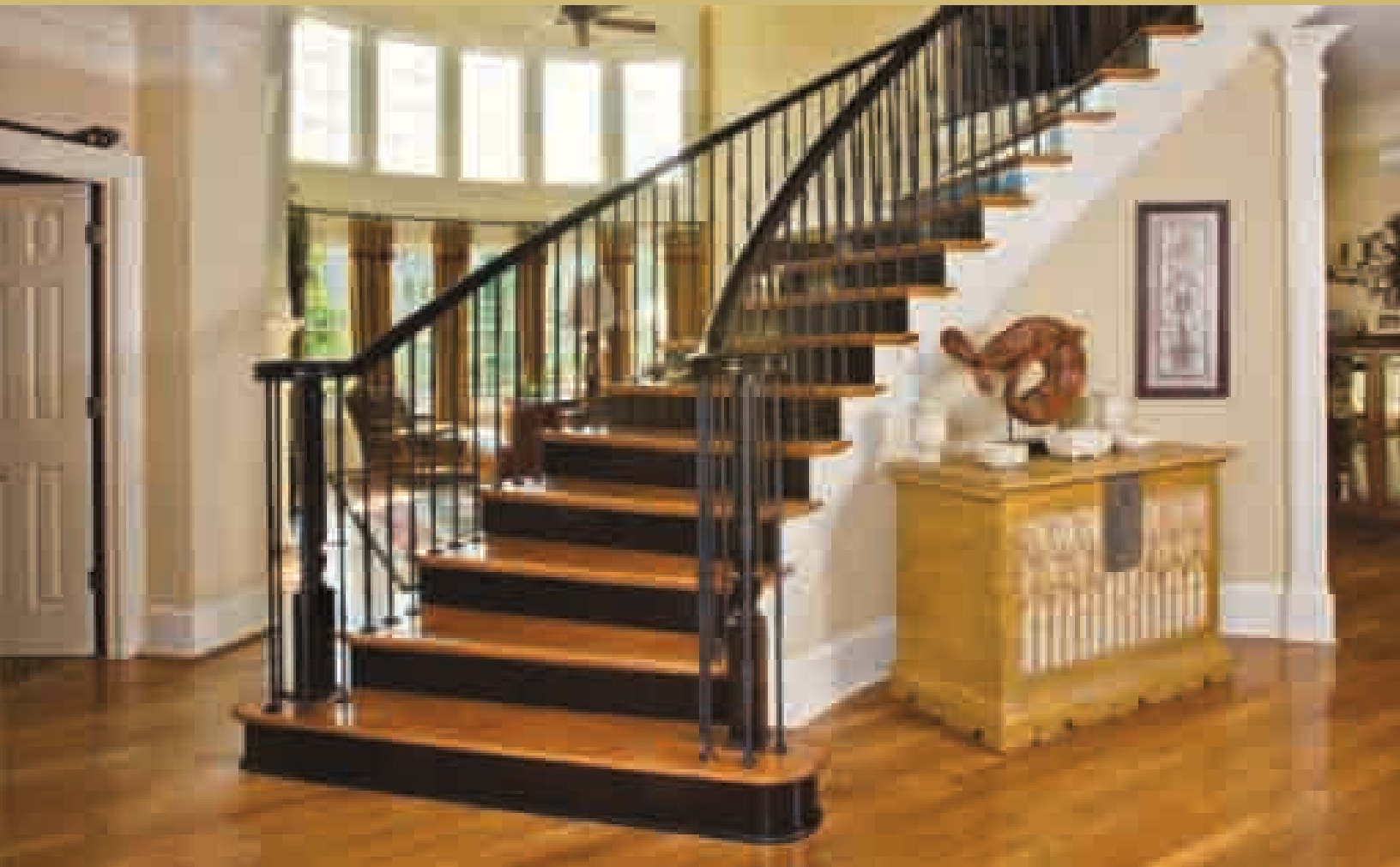
3010 Maple Painted Newel, S1044, S1144, S1244 Satin Black Balusters, 6710 Maple Painted Bending Rail
