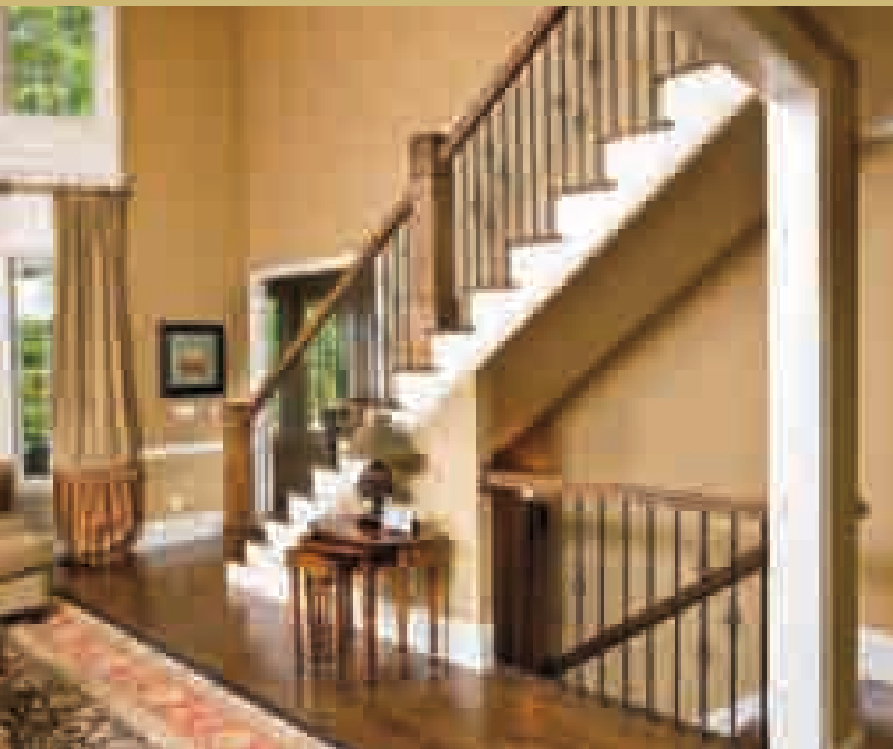
4094 Oak Box Newel, TW Full, BAS144, BAS244 Satin Black Balusters, 6710 Oak Handrail
