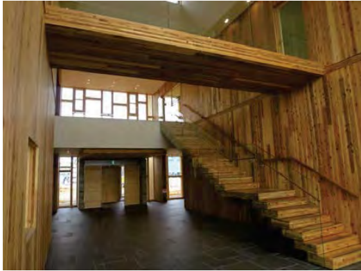
Photo ii: Building using CLT (Kochi prefecture)
