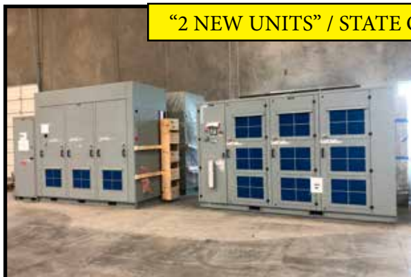
2) SIEMENS SINAMICS PERFECT HARMONY GH180 TYPE 6SR3, 9000HP GEN 4E-CELL SIZE750A MEDIUM VOLTAGE VARIABLE FREQUENCY DRIVE UNIT, 750 AMP CELL, DIGITAL CONTROLS. INPUT 1274AVAC-3PH-60HZ-370A OUTPUT 0-6600V – 3HP – 0-330HZ –750A (SUPPLIES VARIABLE VOLTAGE AND FREQUENCY TO OUTPUT DRIVES)
