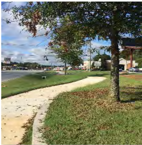
SR-58 multi-use path as constructed.
