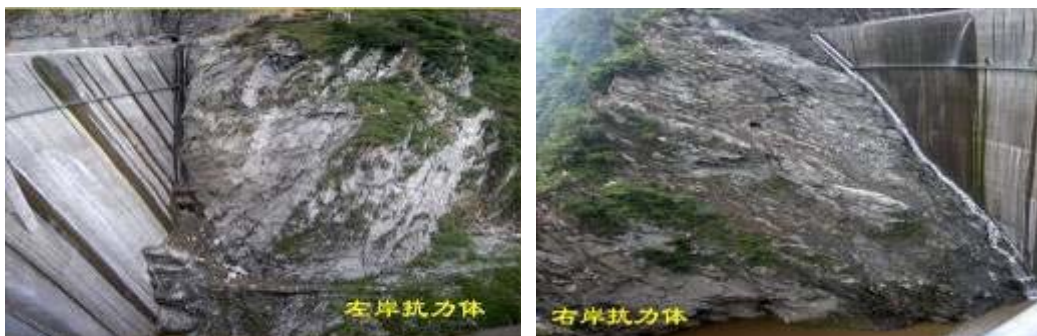
Photo 2. Dam abutment resisting force body is almost well after Wenchuan earthquake
