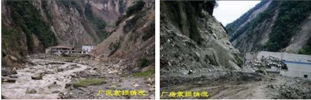
Photo 3. The earthquake damage of the powerhouse
