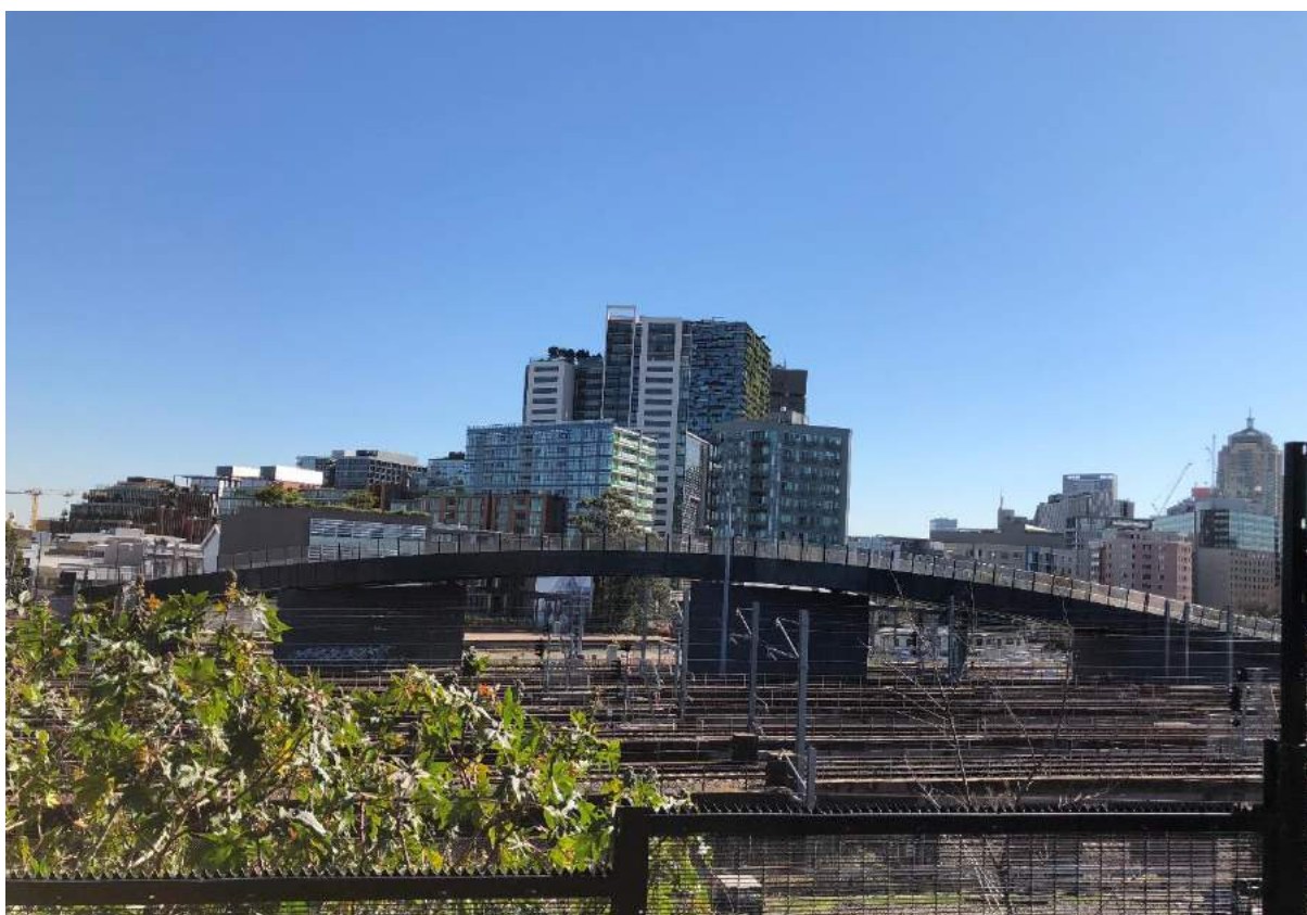
Figure 16 Sydney Yard Access Bridge (SYAB)
