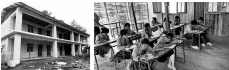
Figure 18: Picture of new School building rented for a bank while student where compelled to study in temporary shelter that was followed by protest from community. By measure of comfort and ventilation and temperature control, the temporary structure might have been a more preferred space for students thought. THT, June 17, 2018 (Asar 3, 2075)
