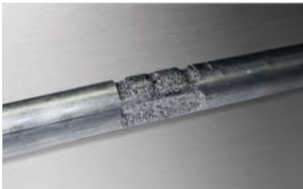
Crevice corrosion formed under a regular plastic clamp
