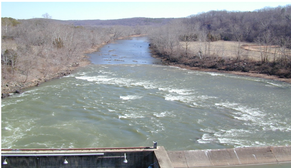
Photo 3. Leesville Reservoir tailrace following power generation.
