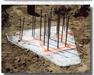
When forming below grade structures like a pile cap, Stay-Form can save a considerable amount of time and labor. You have no labor for stripping forms. If rebar or metal is used for bracing, it stays in place. (Wood bracing has to be removed.) Some contractors backfill around the Stay-Form prior to the pour therefore they minimize bracing and prevent a blowout of the form.
