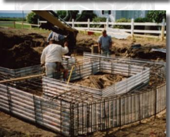
Grade beams are easily formed using Stay-Form and rebar or lumber as bracing. Some contractors prefer to backfill 75 to 90 percent up the grade beam prior to the concrete pour in order to minimize the required bracing. Backfilling acts as the bracing which will stop the formwork from spreading during the pour.
