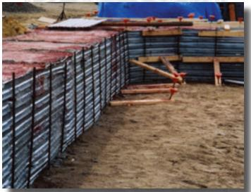
Electrical contractors find it easier to form ductbanks with Stay-Form than with plywood or conventional forming systems. The learning curve to train personnel how to install Stay-Form is quick, and the labor savings are significant due to the fact that form stripping is not necessary.
