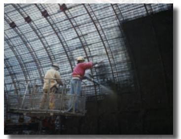
Using Stay-Form as a backstop for shotcrete applications has many advantages. It can be bent to any radius and is easily wire-tied to the reinforcing steel that will form the structure. The open herringbone mesh and V ribs do a great job in catching the shotcrete while minimizing the amount of rebound.
