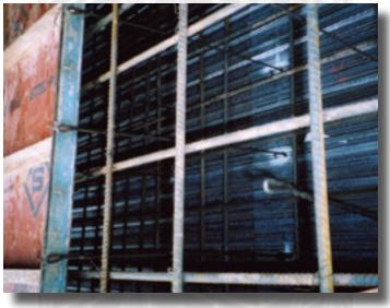
When a contractor has to form a concrete wall within a few inches of an existing structure, Stay-Form is an excellent product. By utilizing Stay-Form with rebar studs, hook ties, and a modular form system, a one-sided form or blindside wall can be constructed. If you do not have the luxury or room to strip formwork, Stay-Form is the right product for the job.
