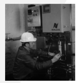
Figure 1: Checking water treatment control system.
