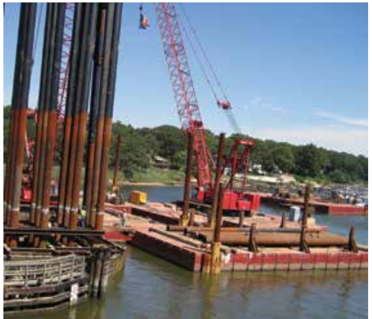
New Jersey Department of Transportation, Brielle, NJ
