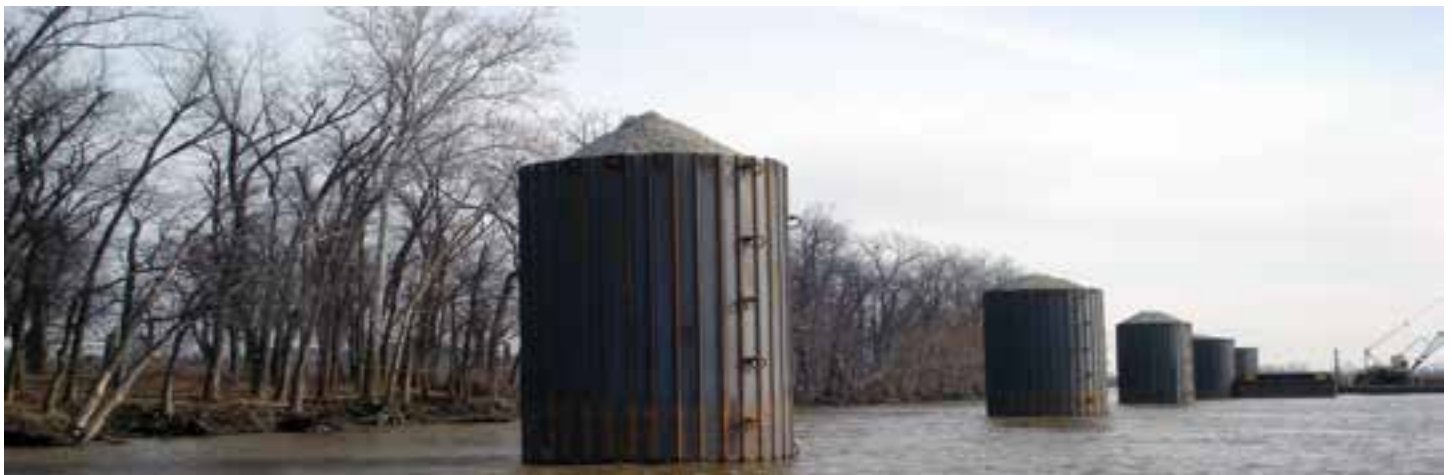
Sitrان Coal Transfer Facility, Mount Vernon, IN
