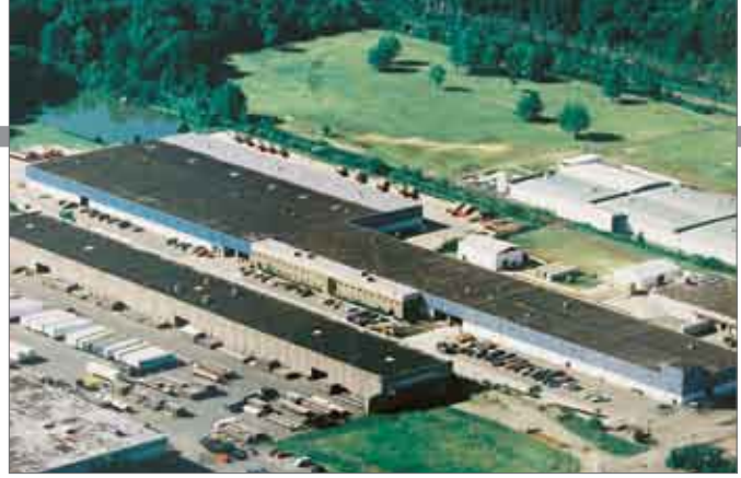
South Plainfield, NJ
