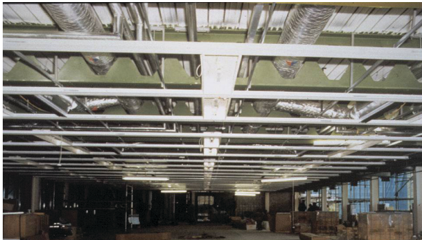
Fig. 2-5. Openings utilized for conduit and HVAC routing.
