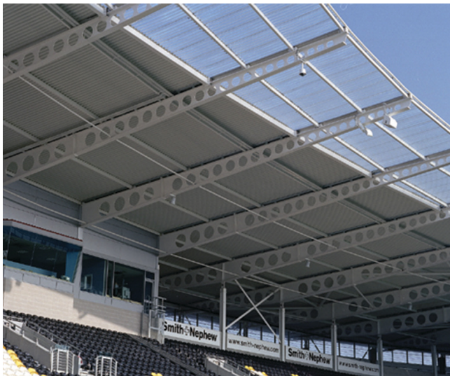
Fig. 2-9. Tapered roof support beams.
