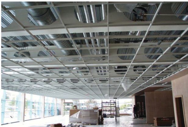
Fig. 2-6. Service integration with ceiling attached to structure.
