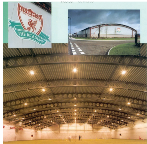
Fig. 2-8. Curved cellular beam roof structure.
