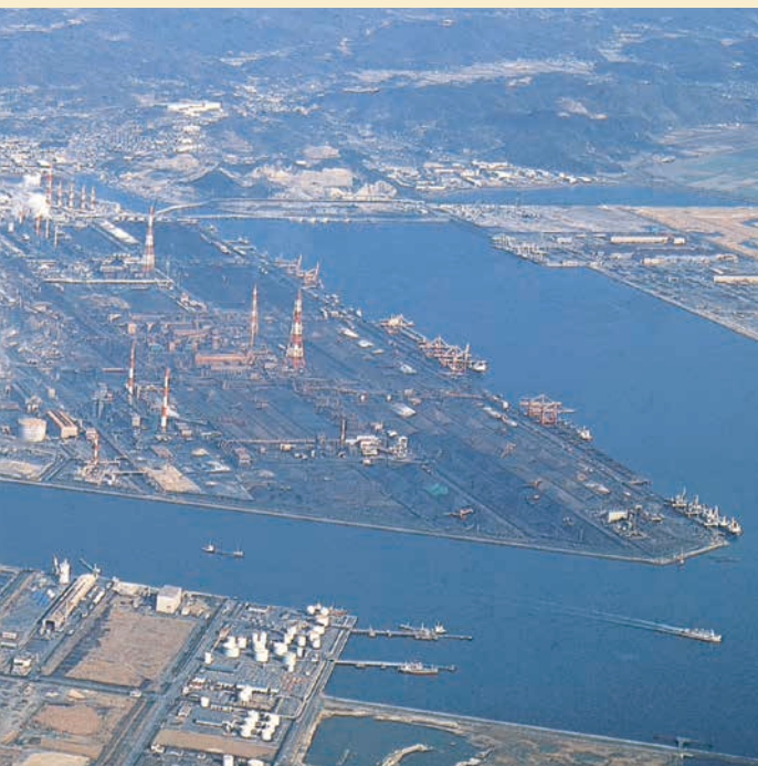
West Japan Works (Fukuyama)
