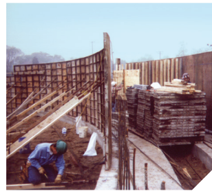
Curved Wall Forms using Steel-Ply
