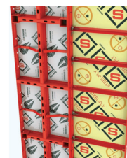
Sym-Ply to Steel-Ply transition
