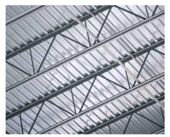
**Steel Joists and Deck**ROOFING AND FLOORING SYSTEMS
