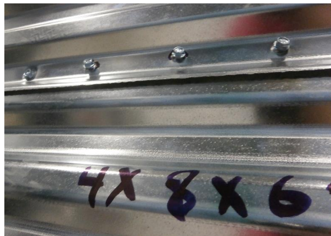
Figure 38 - a. Test 5 failure mode - sheathing connection failure, b. screw failure at bottom track, c. seams screw pull out
