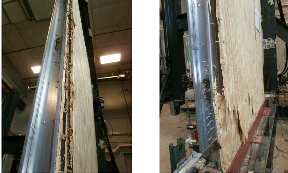
Figure 39 - Test 11 failure mode
