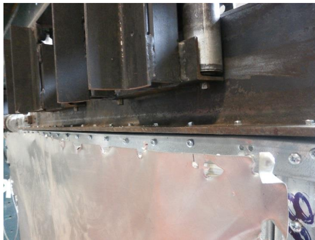
Figure 40 - Test 12 failure mode - sheathing screw pull over at top track
