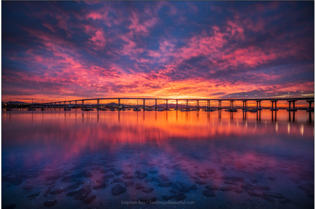
A spectacular sunrise over the Coronado Bridge as seen from Tidelands Park, 11/14/18.
