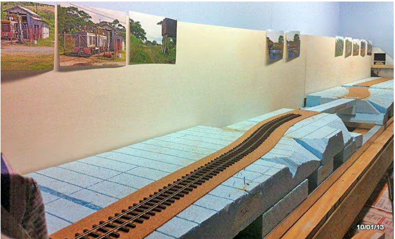
Two modules under construction: the 25mm Queblok Aluminium framing and extruded polystyrene define the layout's dimensions, with the joint between modules visible to the right of the photo. The extruded polystyrene has been roughly shaped and track location determined. Steve Pettit photographer.
