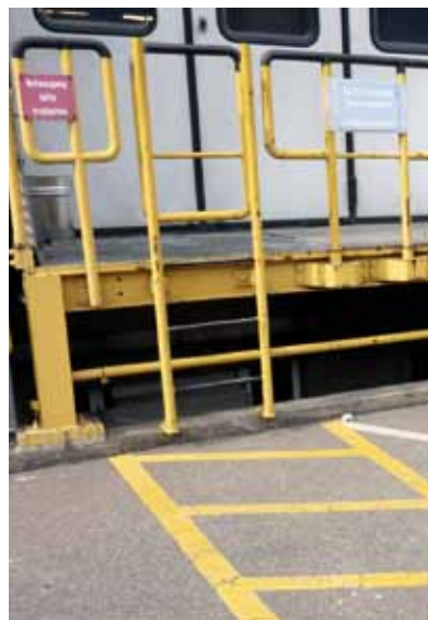
Escape routes must not be blocked
