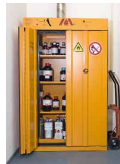
Safety cabinet for flammable liquids
