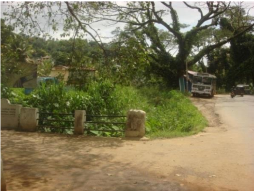
Figure 4. Red Culvert Upper
