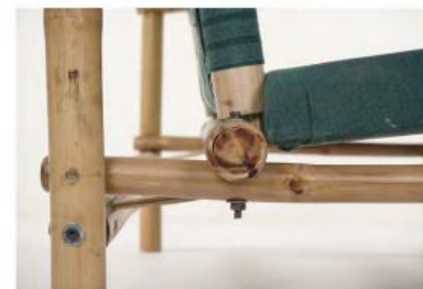
L Split Bamboo Joinery Detail
