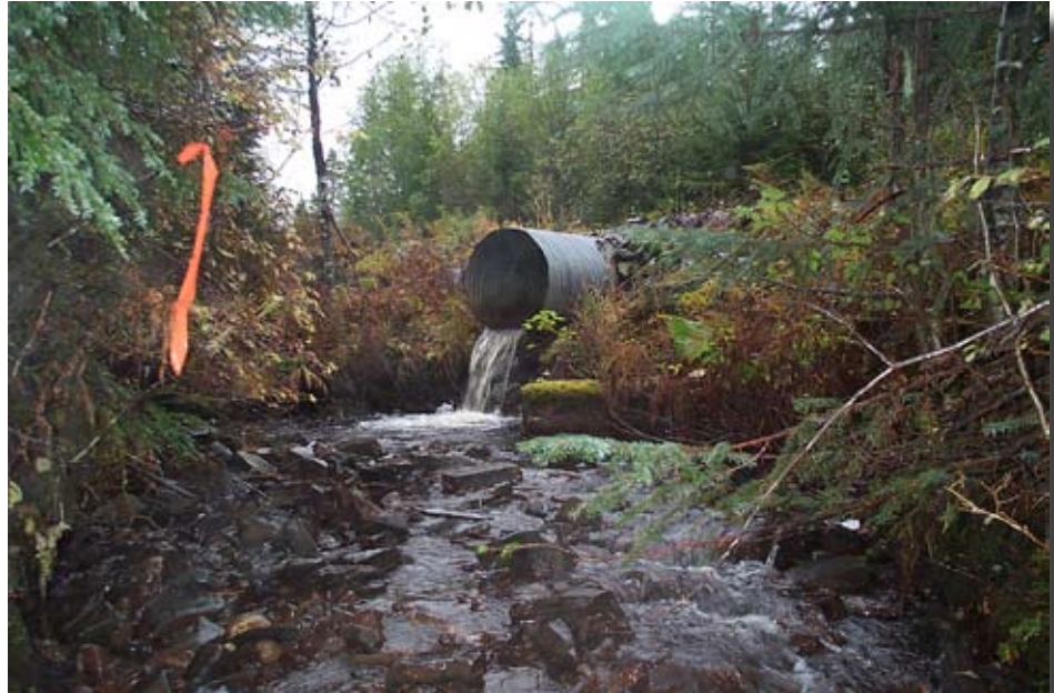
Figure 6.14—Looking upstream at outlet of existing pipe, road 6245. Photo: Chinook Engineering.
