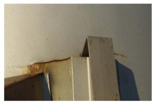
Figure 5. Crack A<sub>1</sub>
