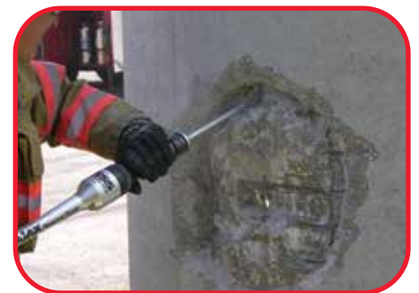
Breaching Concrete
