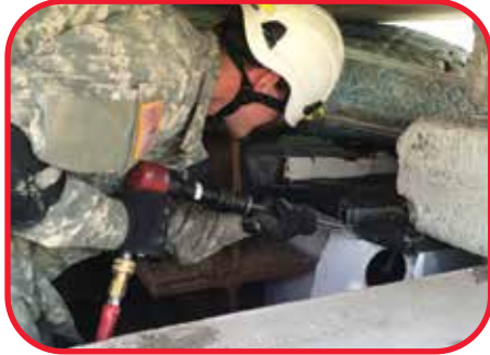
Cutting through dryer in collapse
