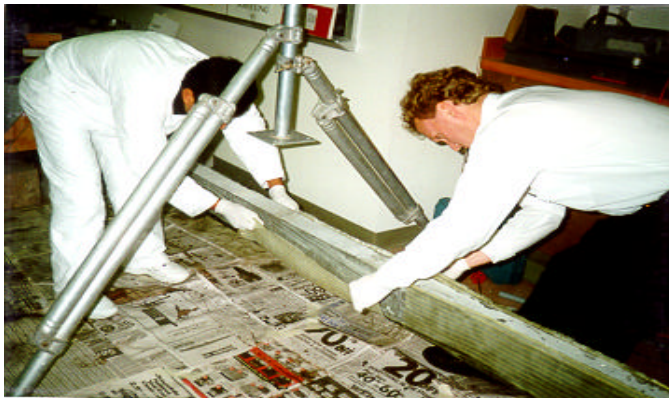
Figure 4 – Students applying fiberglass-reinforcing mesh to beam
