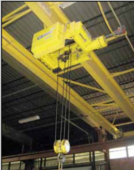
(1 OF 2) ABLE HOWE 5-TON RF REMOTE CONTROL DOUBLE GIRDER BRIDGE CRANES
