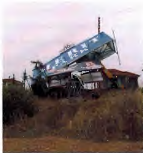
Figure 1.7. Signboard fall due to wind storm
