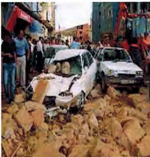
Figure 1.6. Damages due to fallen minaret
