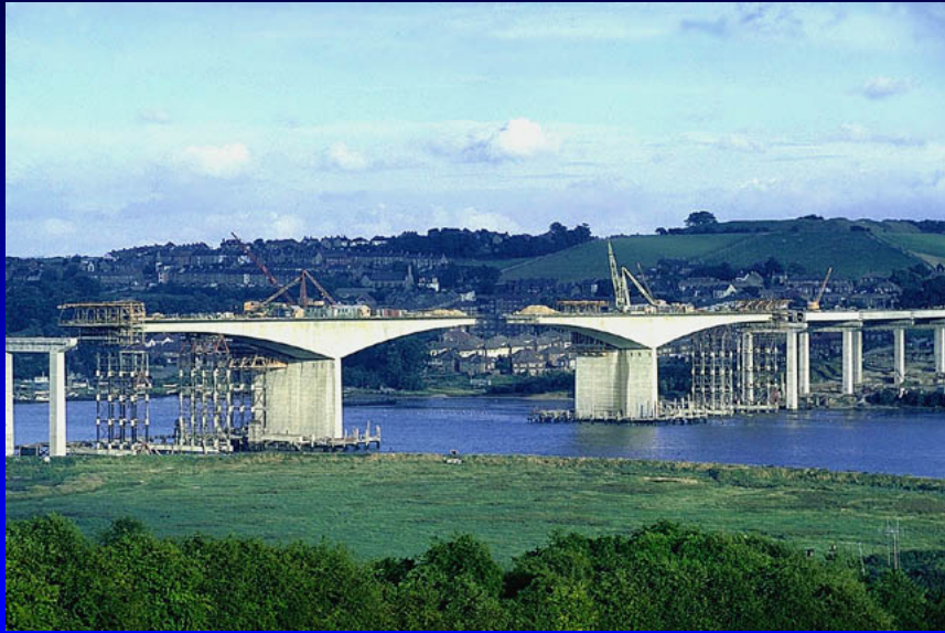
Cantilever Bridge – Variable Cross-Section
