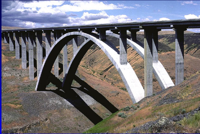
Selah Creek, Yakima, Washington
