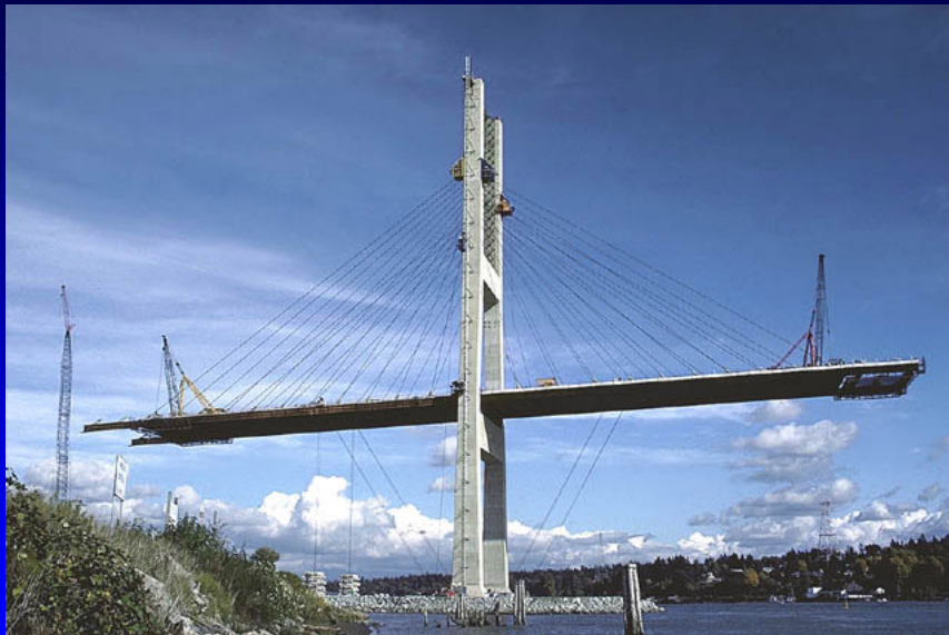
Alex Fraser Bridge – Cable-Stay Construction
