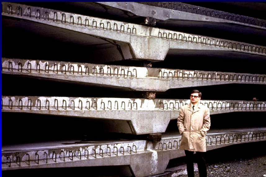
Variable Section Precast Members
