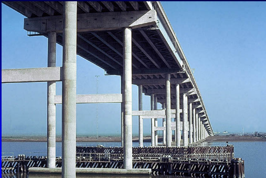
Bridge Frames Supporting Precast Concrete and Steel Beams
