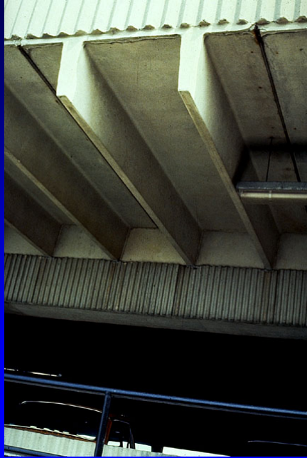
Double-Tee Precast Roof Beams
