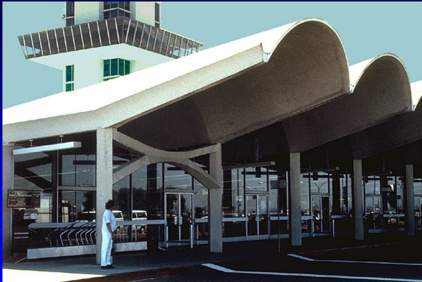
Barrel Shells, Oakland Airport
