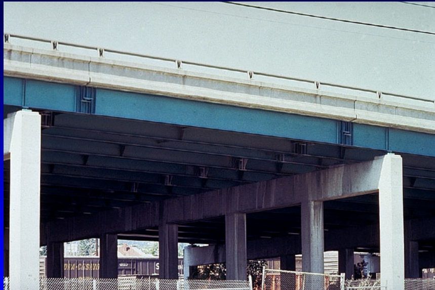
Rigid Frames – Overpass
