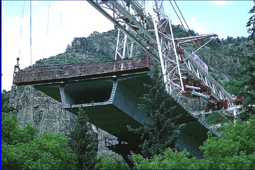
Post-Tensioned Segmental Bridge (I-70, Colorado)
