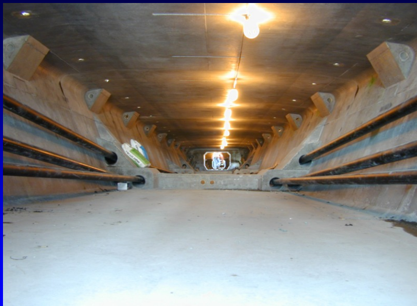
Interior of Box Girder
