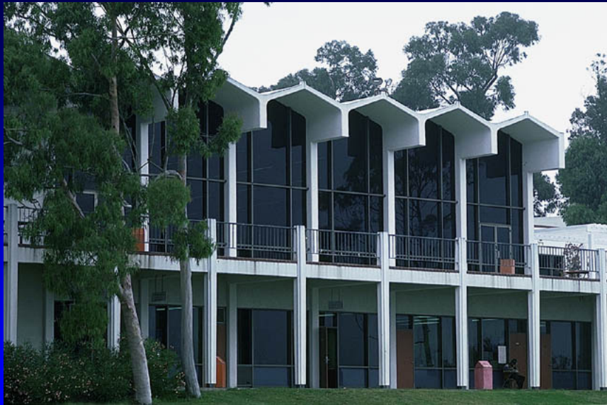
Y-Shaped Precast Roof Beams
