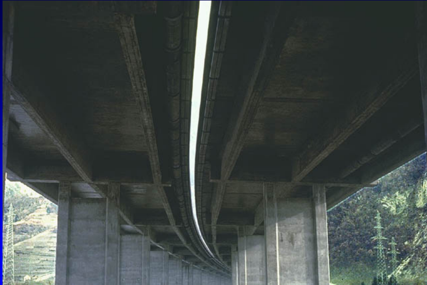
Slab and Beam Bridge
