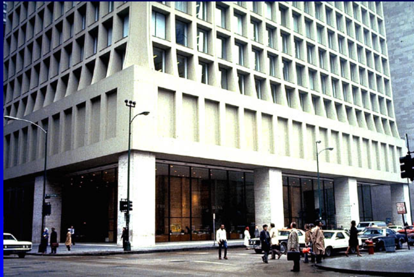
Deep Beam (Transfer Girder), Chicago
