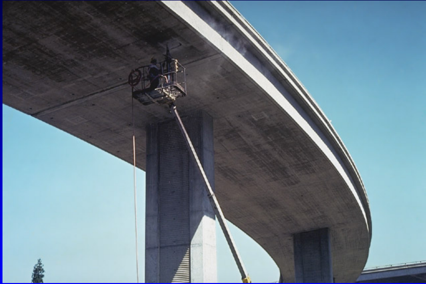
Flat Slab-Column Bridge
