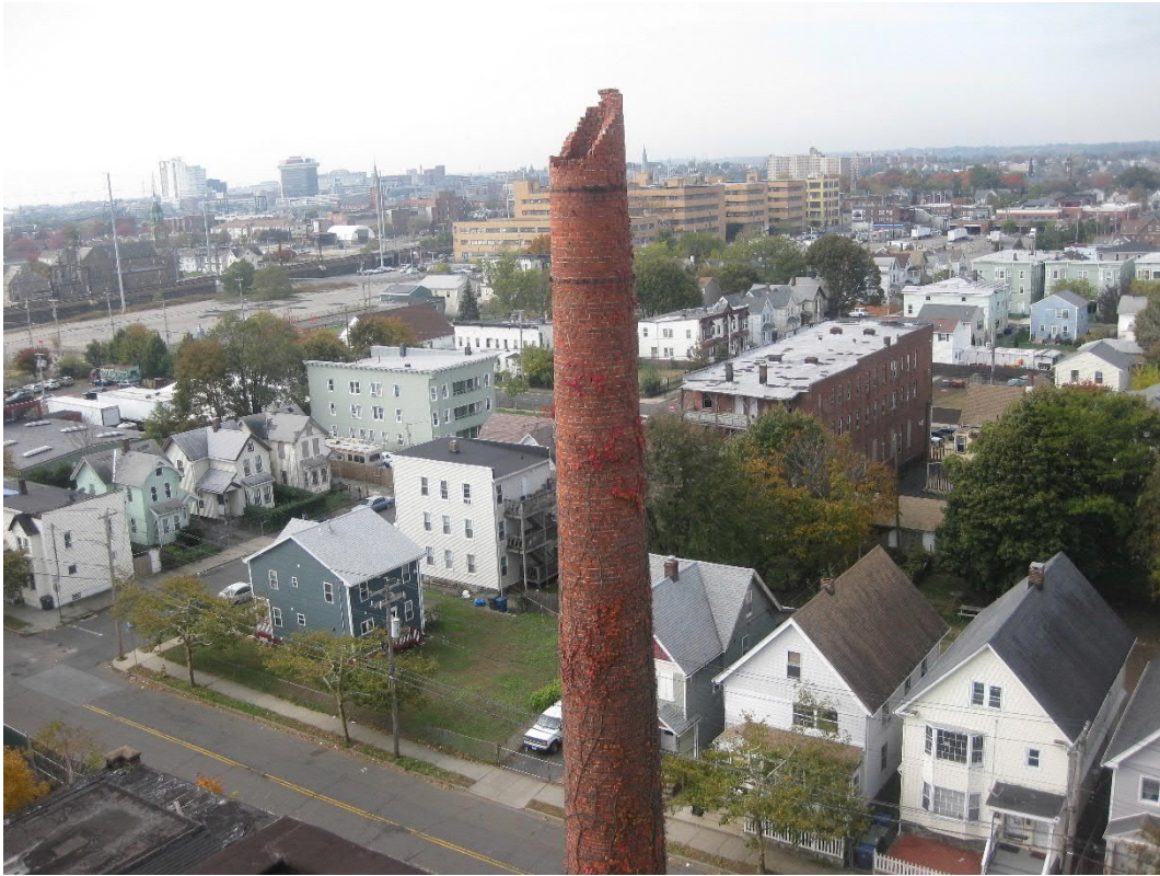
Photo #24 – Upper portion of stack
