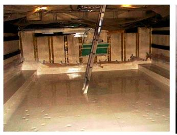
Photo 5- Battery Compartment- pitting corrosion
