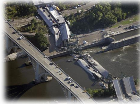
I-35 bridge collapse (Minneapolis, US, 2007) Need of repair – failure of gusset 13 killed +145 seriously injured
