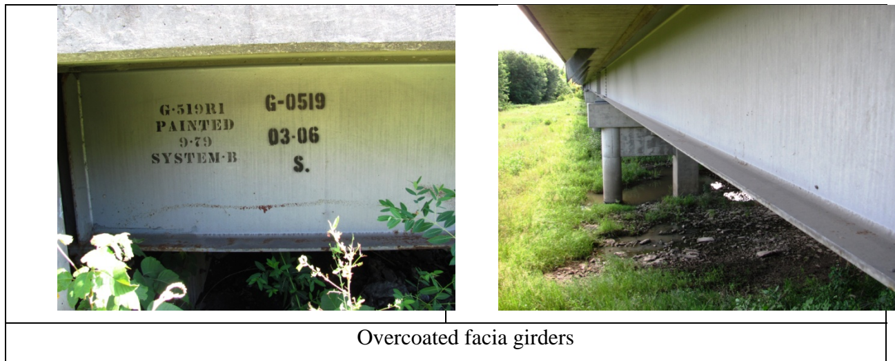
Figure 4.4 Example of System S Overcoating with Good Performance.
