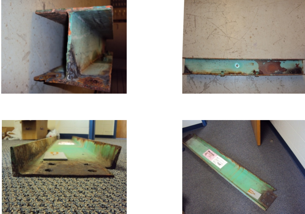
Figure 4.11 Old Decommissioned Bridge Components.
