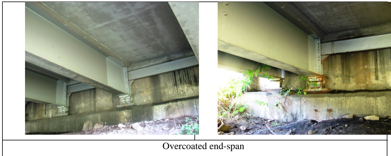
Figure 4.5 Example of Interior Beam-ends with System S Overcoating.
