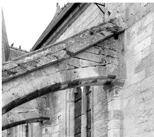
Figure 7. Sliding near the head of a flying buttress at Saint-Julien in Royaucourt (photo Tallon)
