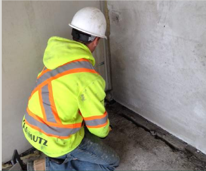
Caulking and second coat of paint
