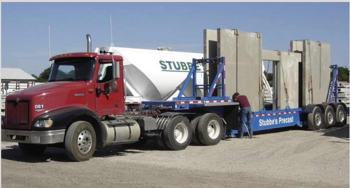
Panels are loaded on trucks and shipped to site.
