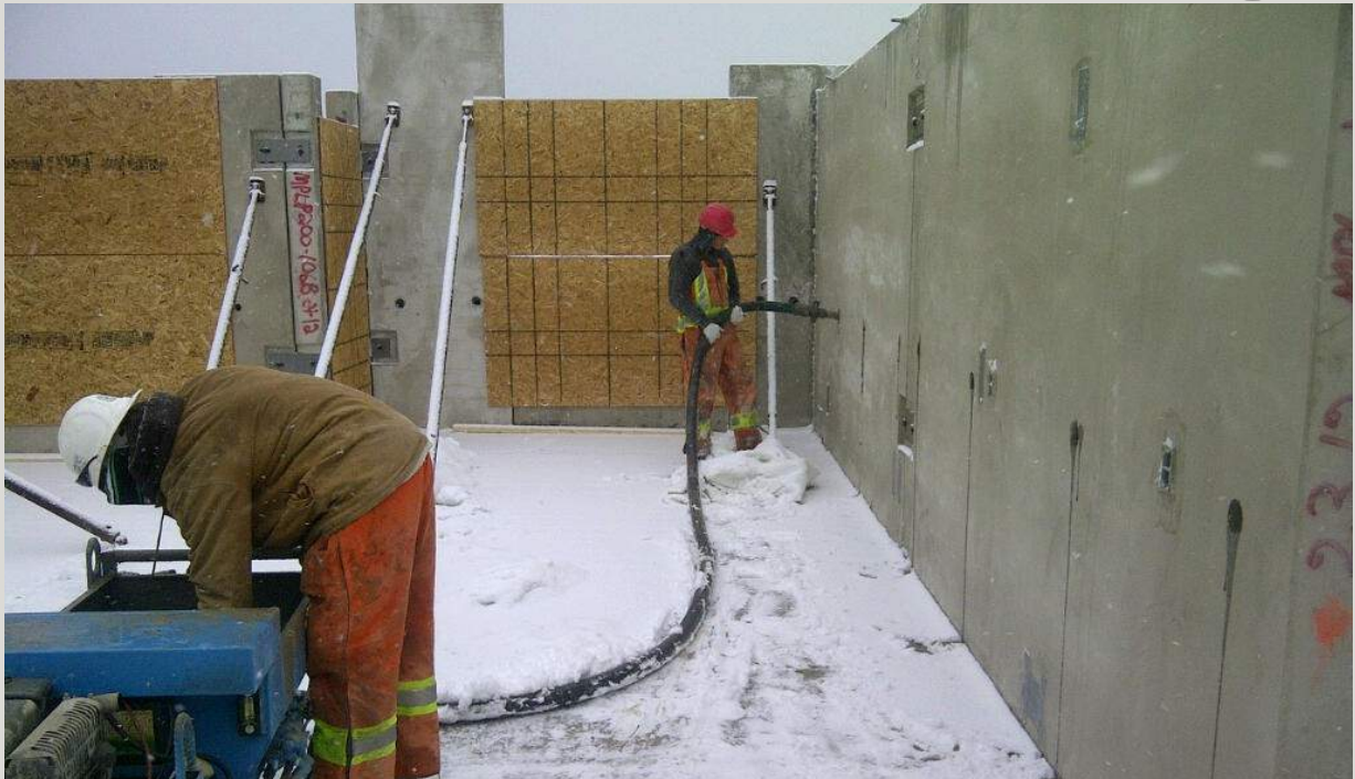
Filling of grout tubes.
