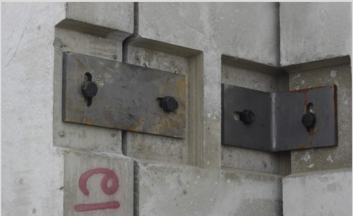
Panel to panel connections are completed.
