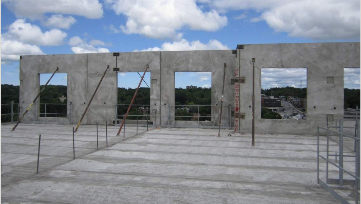
Panels are temporarily braced until connections are completed.
