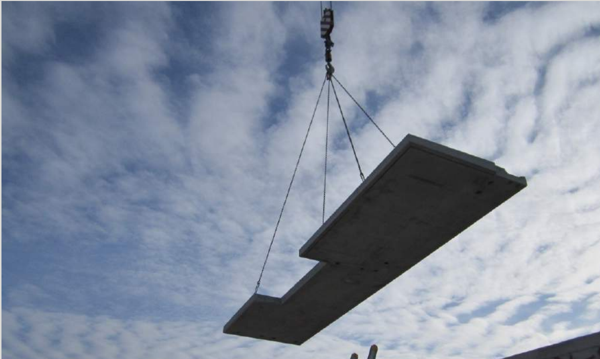
Panels are lifted to the work surface.
