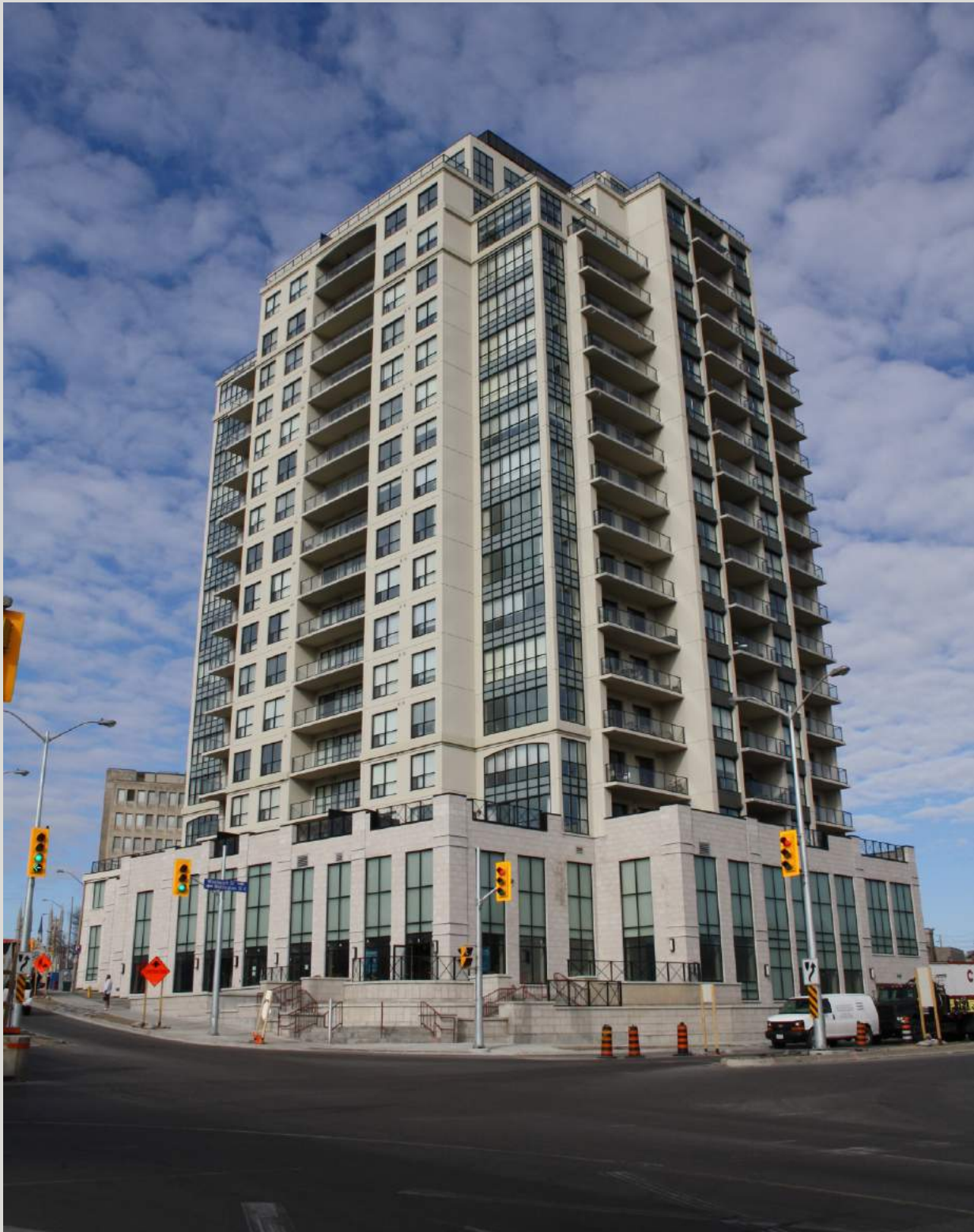
RIVER HOUSE CONDOMINIUMS 18 Story precast condominium for Tricar Location – 150 Macdonell St., Guelph, Ontario
