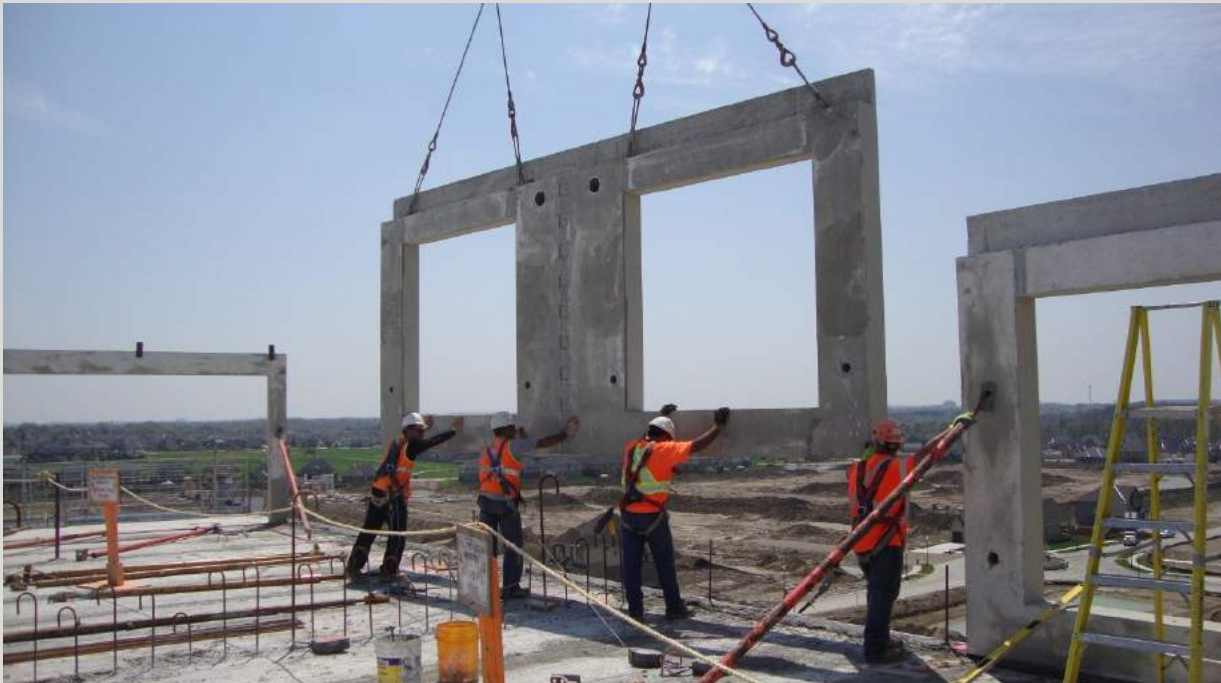
Panels are set into place.
