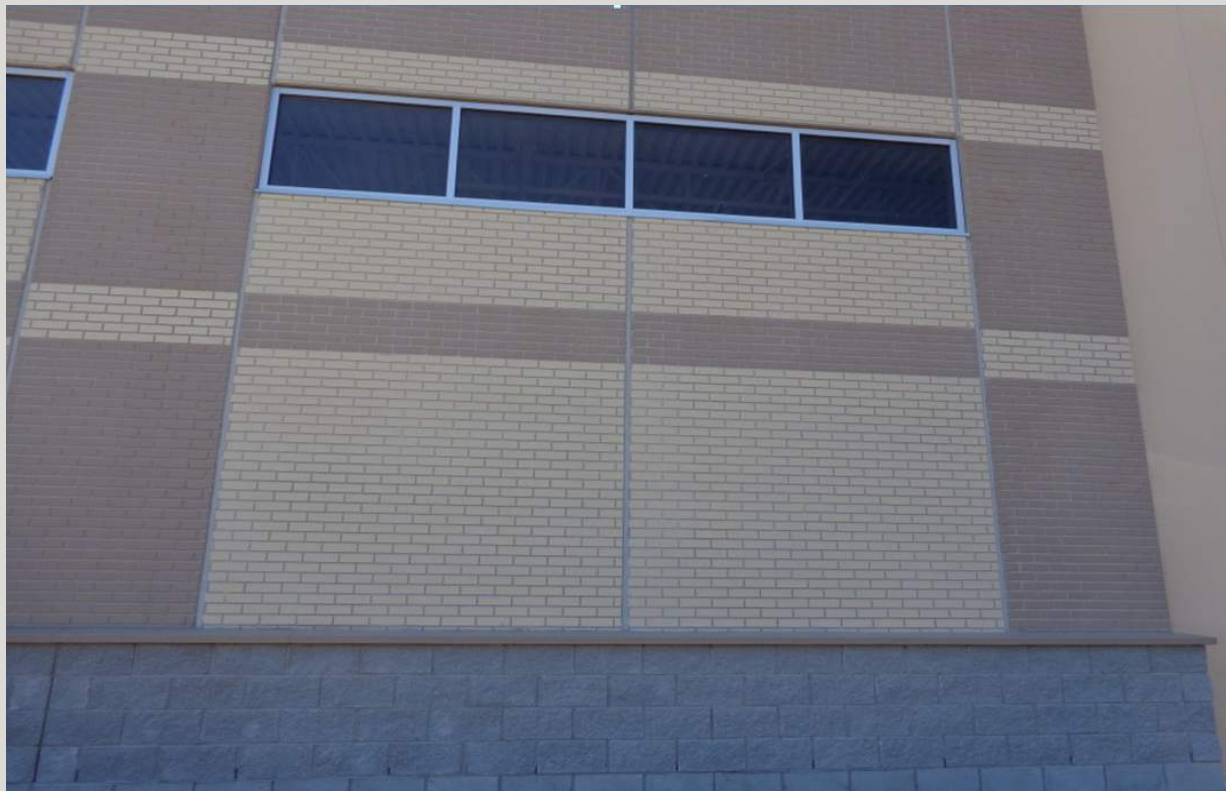
Mold Liner and Paint
