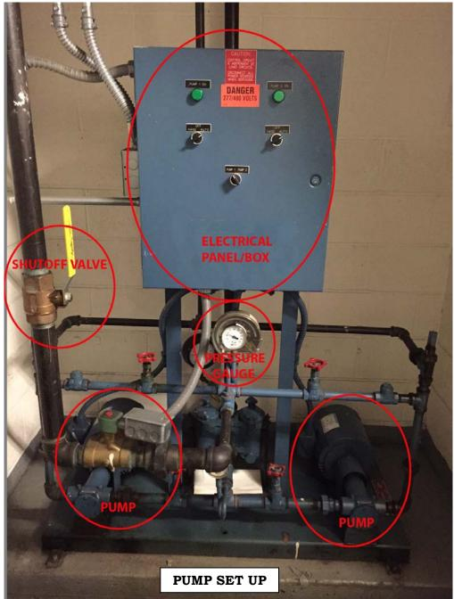
pumps will provide 100% of the maximum required flow. If the load is reduced, say in a burner, one pump may be adequate and the electrical demand will be reduced.
