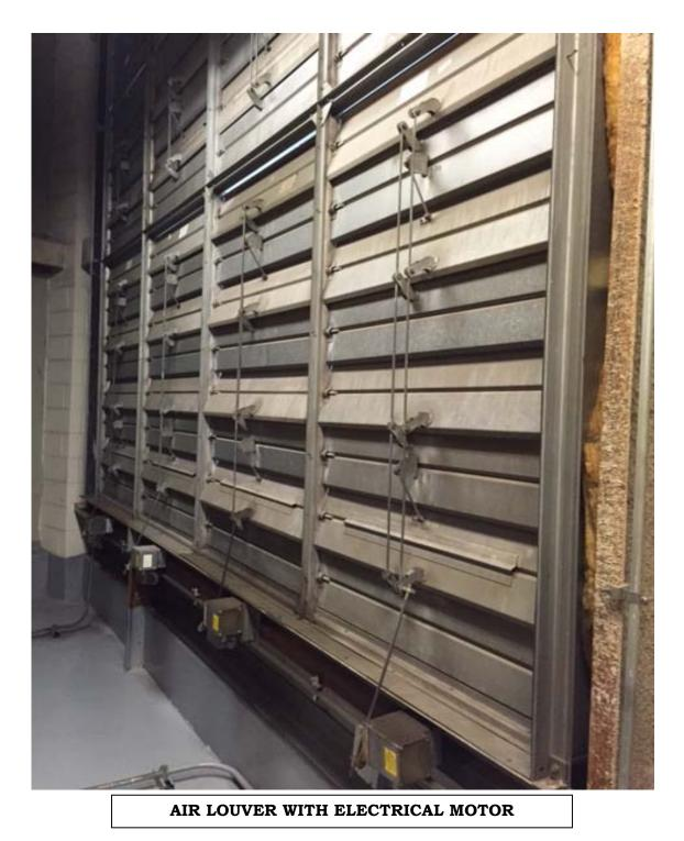
Environmental conditions are critical; the air louver seen above helps to regulate the temperature in the room for the generator, and also helps to regulate in extreme weather conditions.
