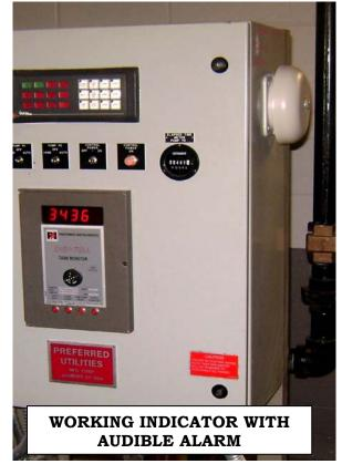
of the tank or the control in the tank. The P-98 Certificate of Fitness holder must take notice of the alarm or bells and take appropriate action. For example, if an day tank alarm goes off – in addition to corrective action it must be logged in the logbook.
