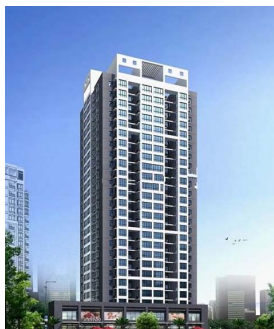
Fig.1 Antie high-rise residential and commercial complex building
